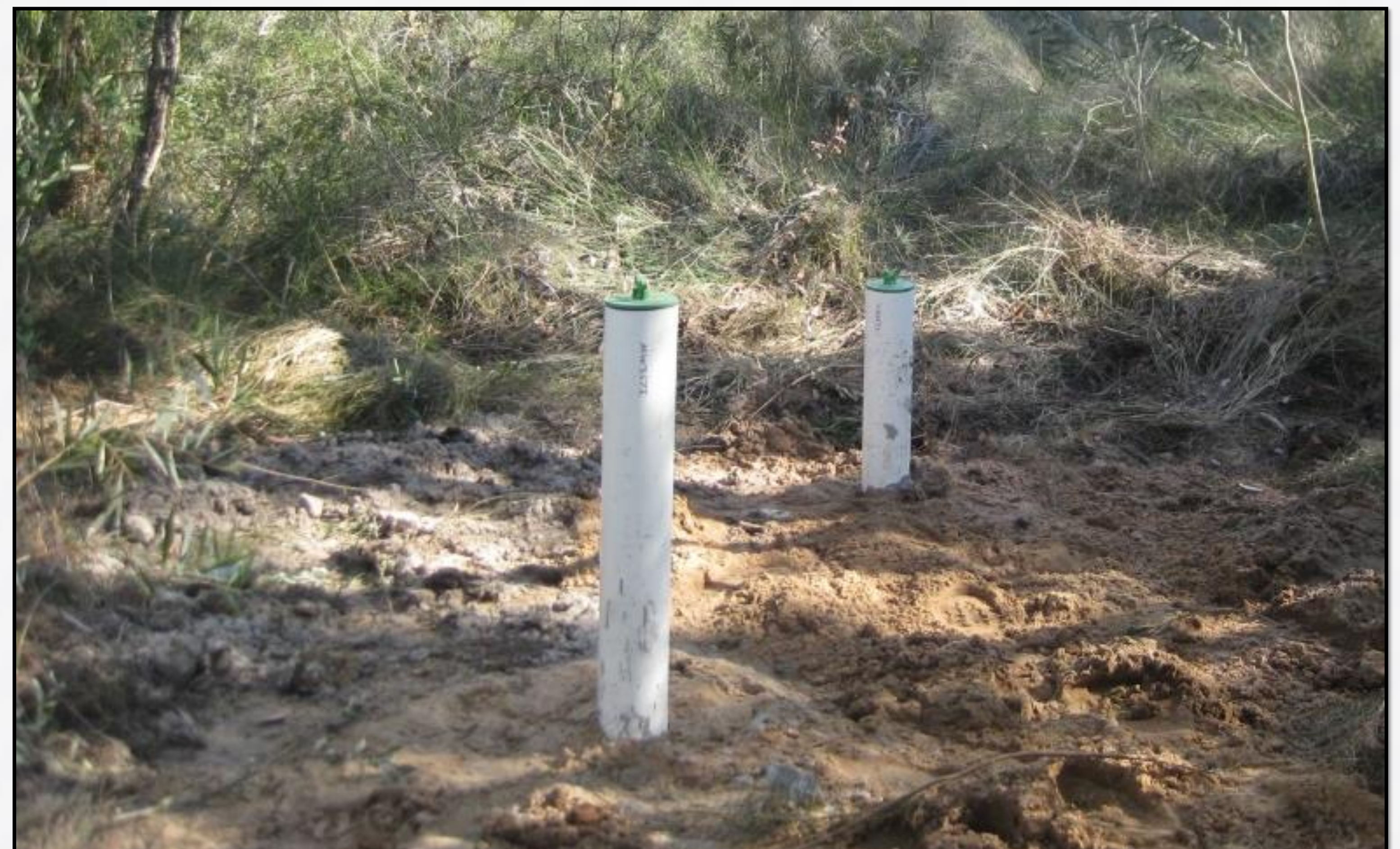
Southern boundary groundwater extraction wellfield
