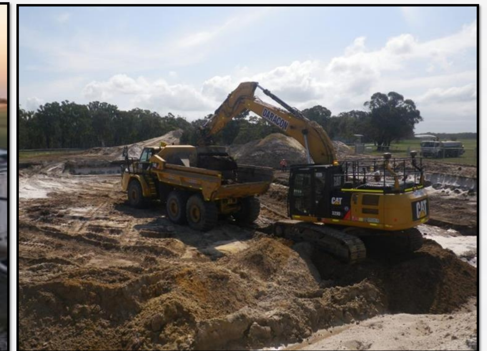
Soil excavation from former fire training area
