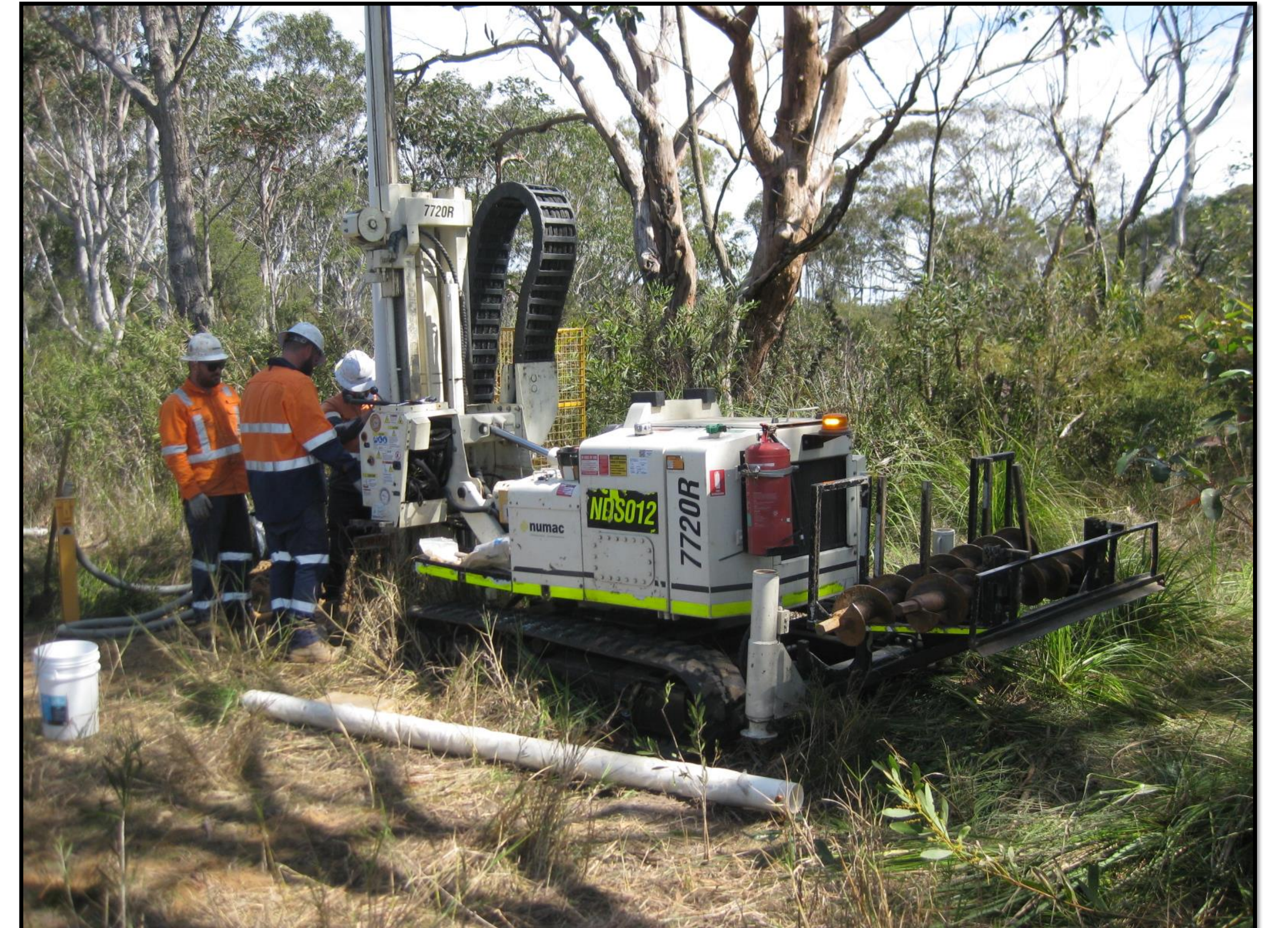
Extraction well installation in Western Region completed in September 2023
