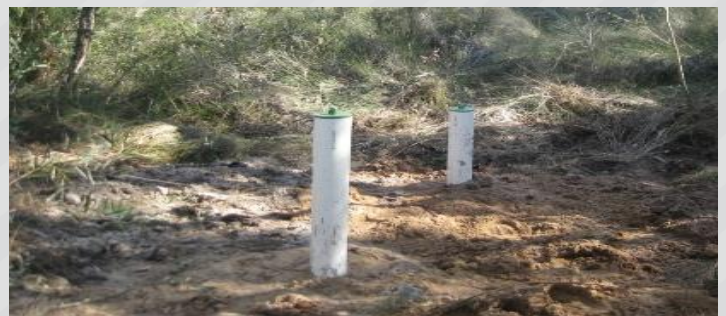
Relocated groundwater extraction wells on the southern base boundary
