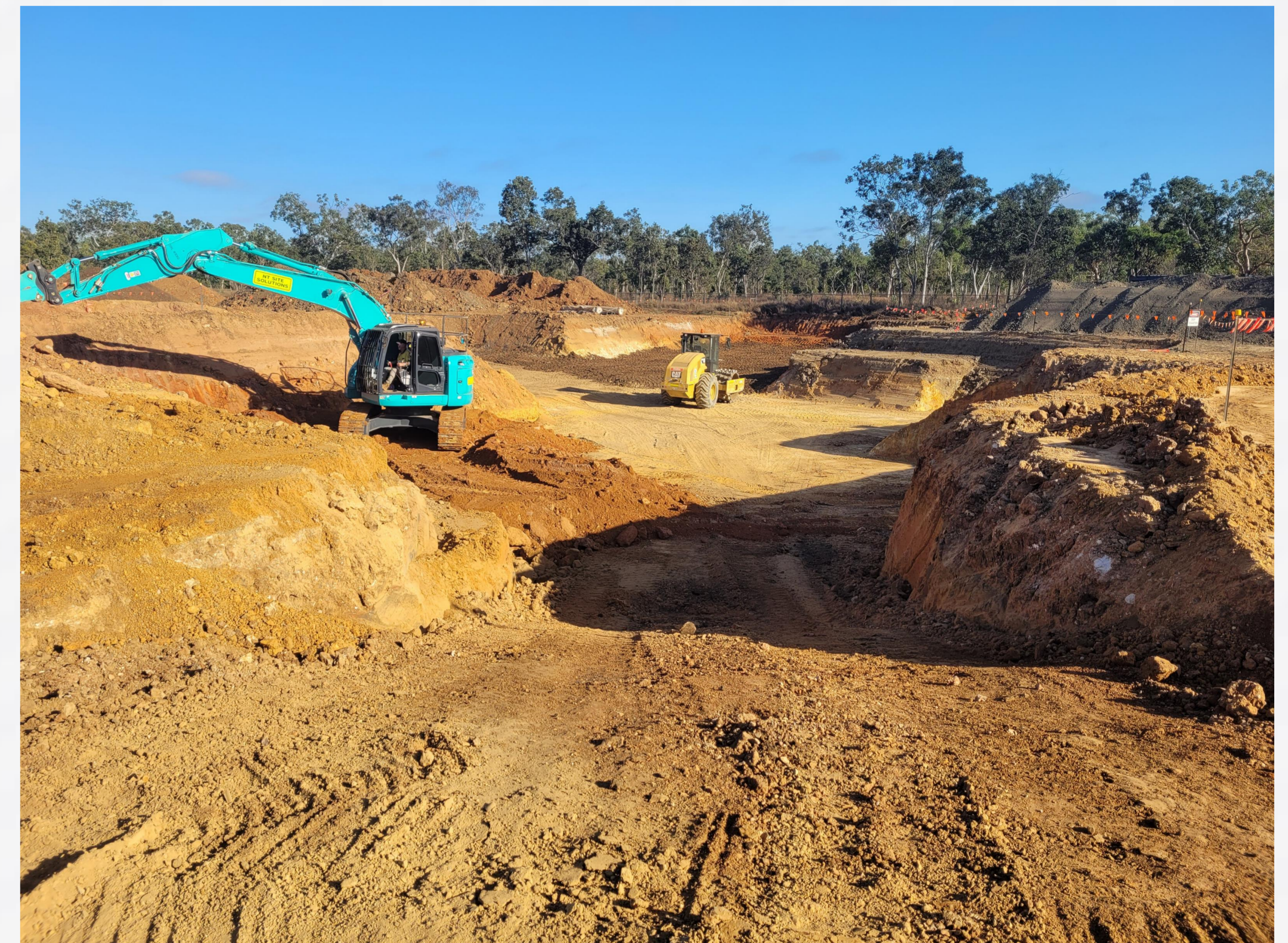
Soil remediation works at the fire training area.
