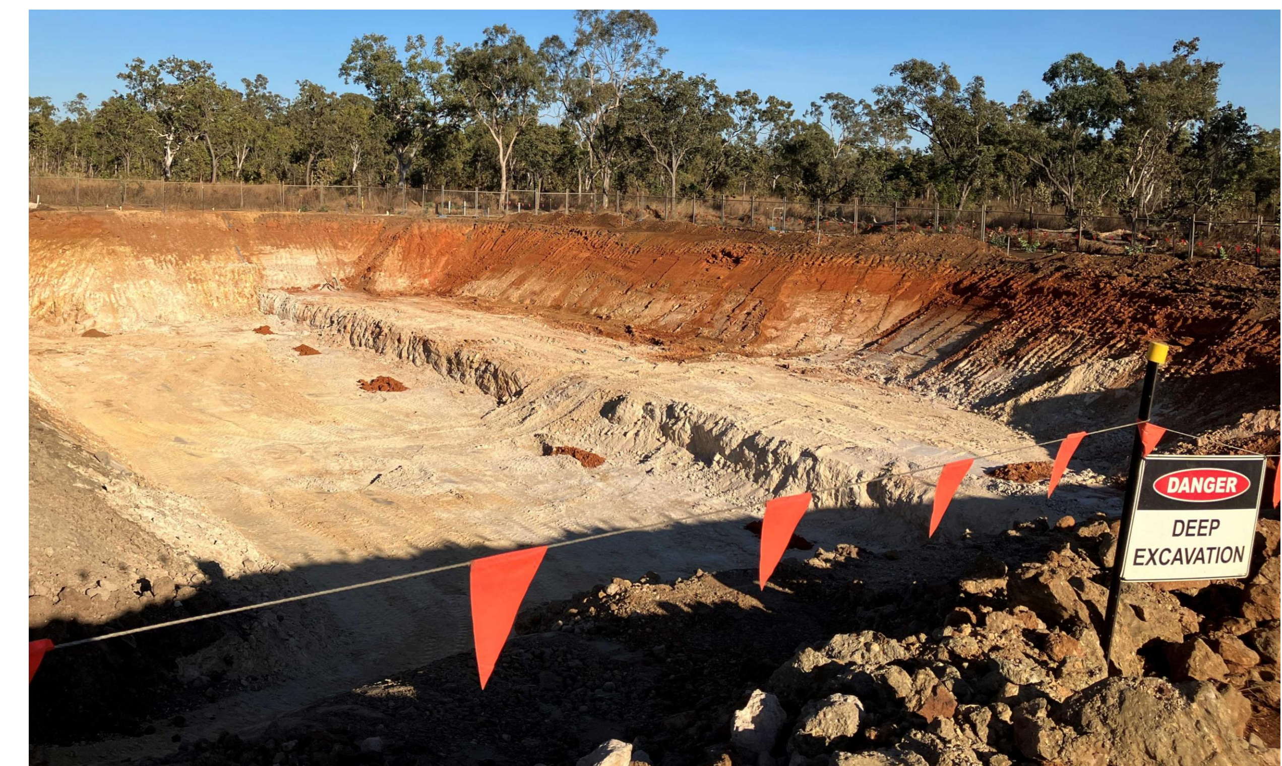
Soil remediation underway at the fire station area
