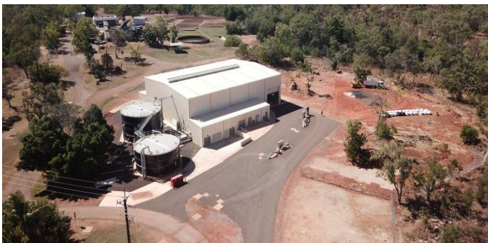
Katherine water treatment plant.
