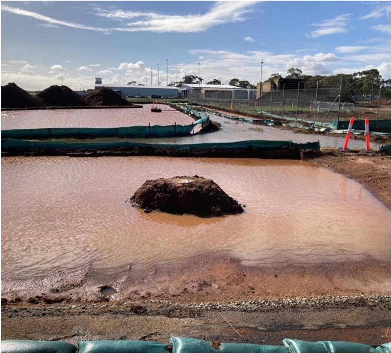
Figure 1 P9 excavation 6 June 2022
