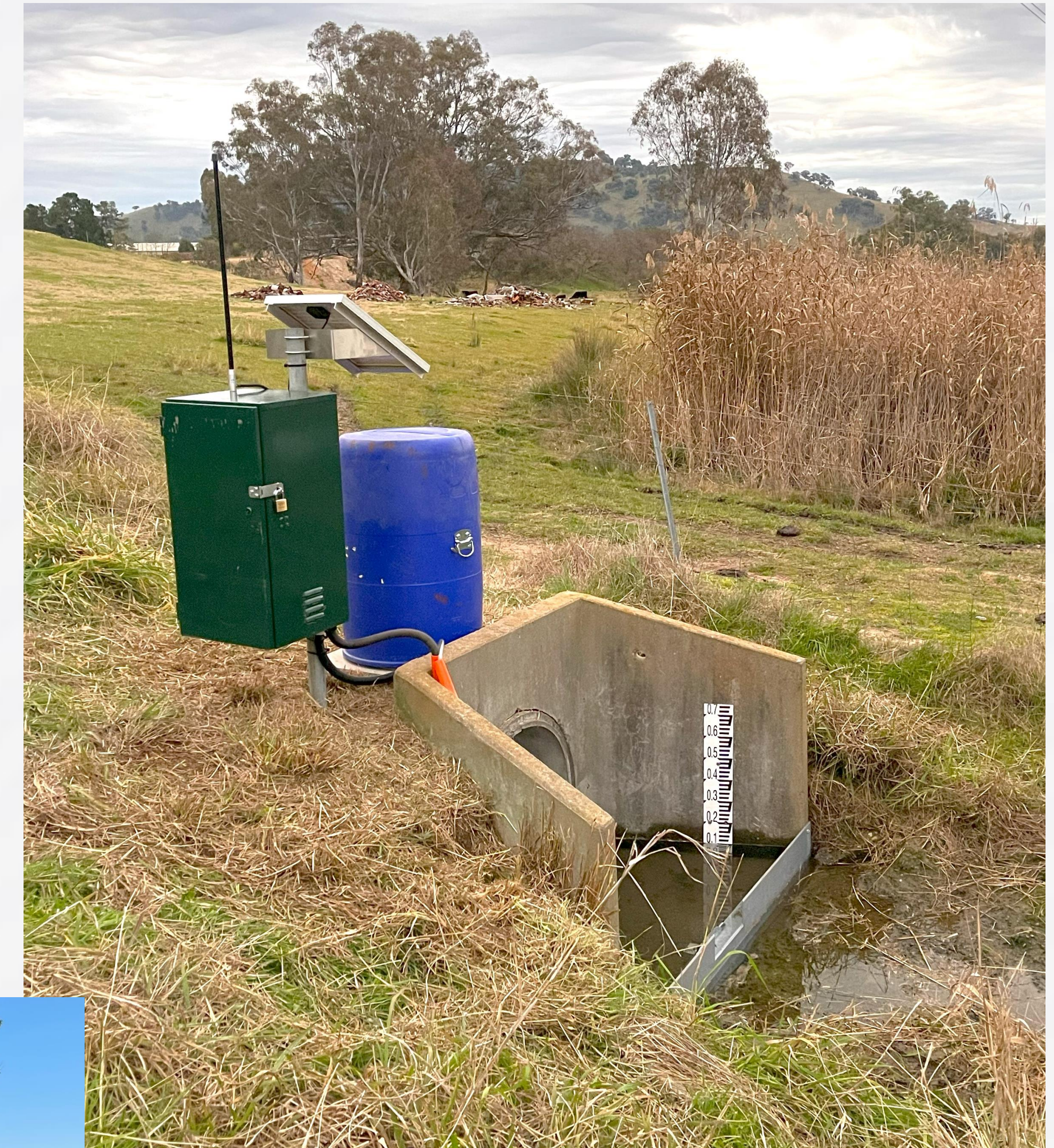
Above: surface water monitoring equipment installed within an on base drainage channel..
