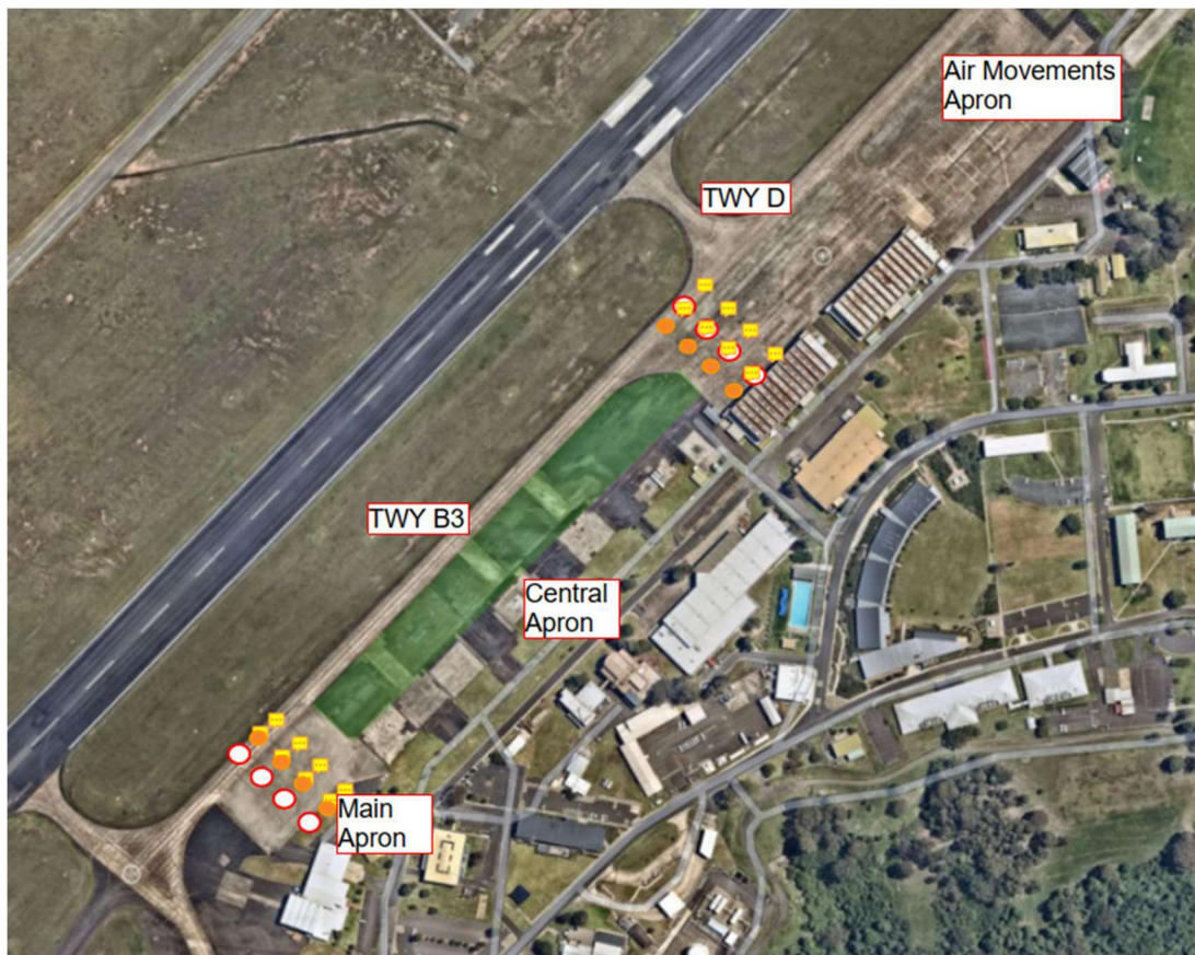
Figure 5 - Central Apron Closure for AC Works
