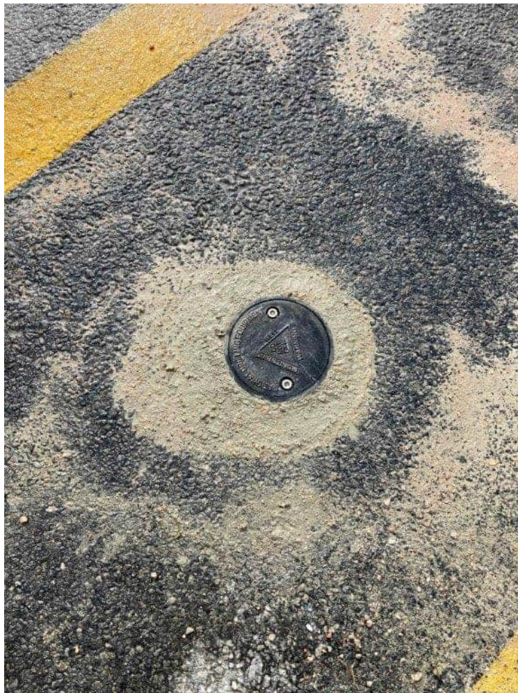
Plate 1 Replacement gatic cover at MW016
