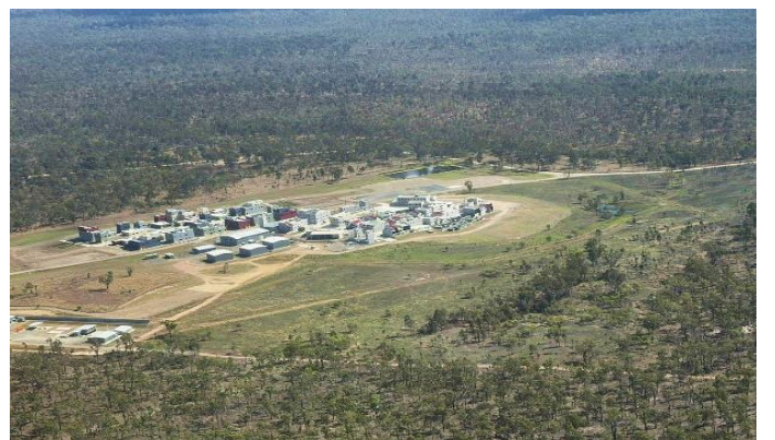
Above: Aerial view of Raspberry Creek Urban Operations Live Fire / Training facility
