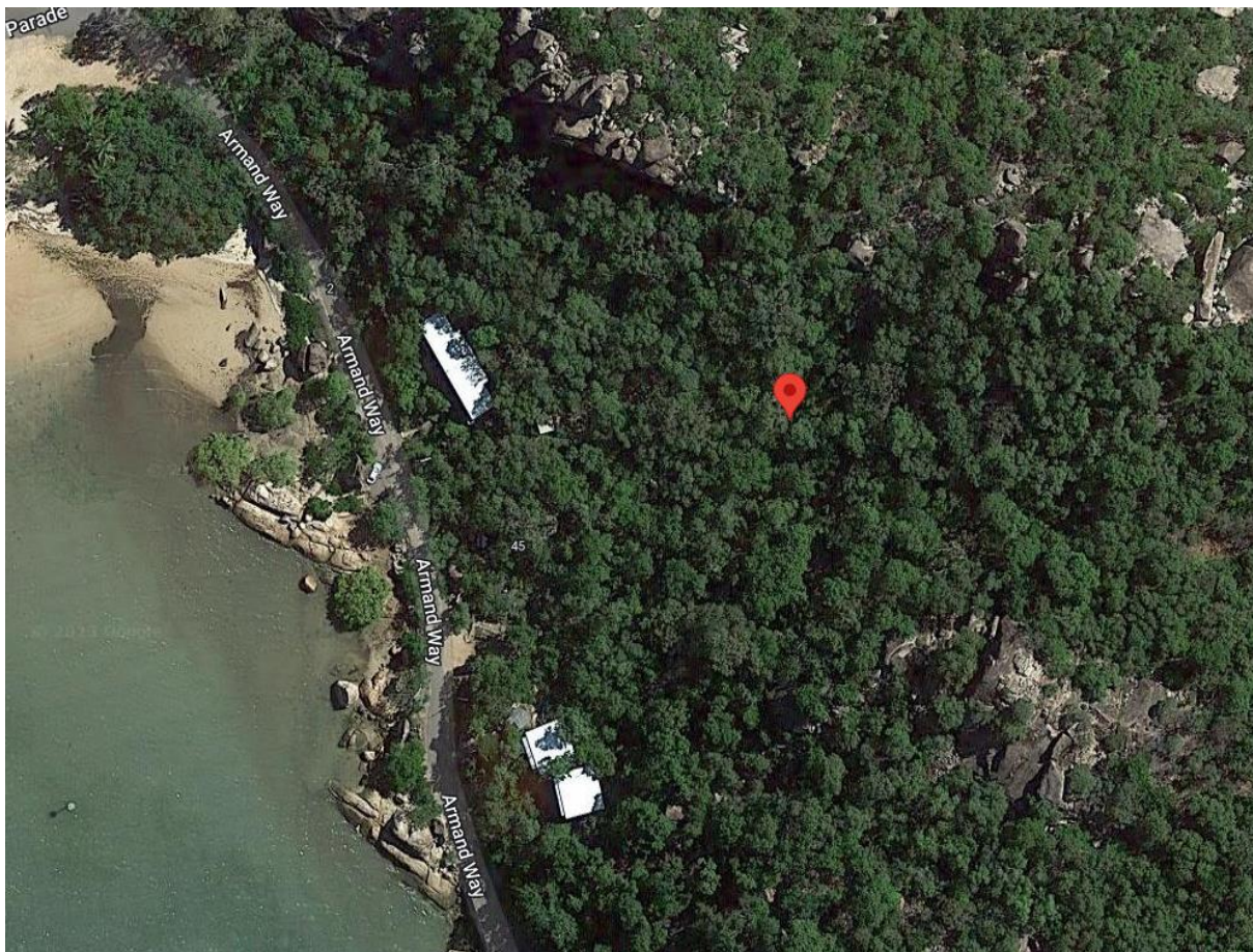
Aerial image of former holiday apartments at Magnetic Island 33-49 Armand Way, Arcadia, Magnetic Island QLD
