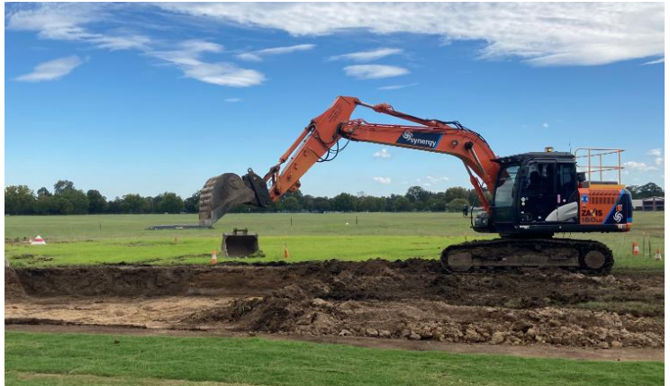
Image: Excavation works at RAAF Base Richmond
