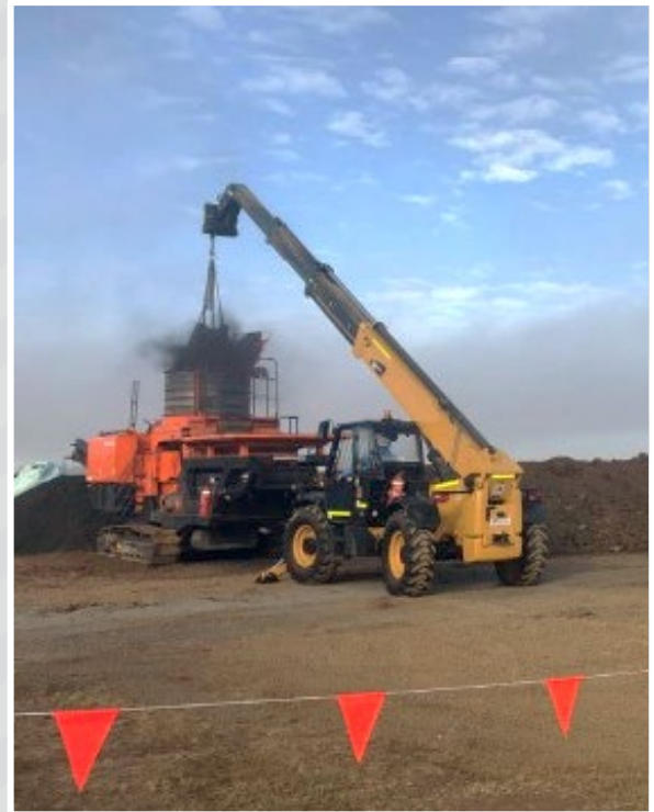
Image 1: Remediation works at Former Fire Training Area
