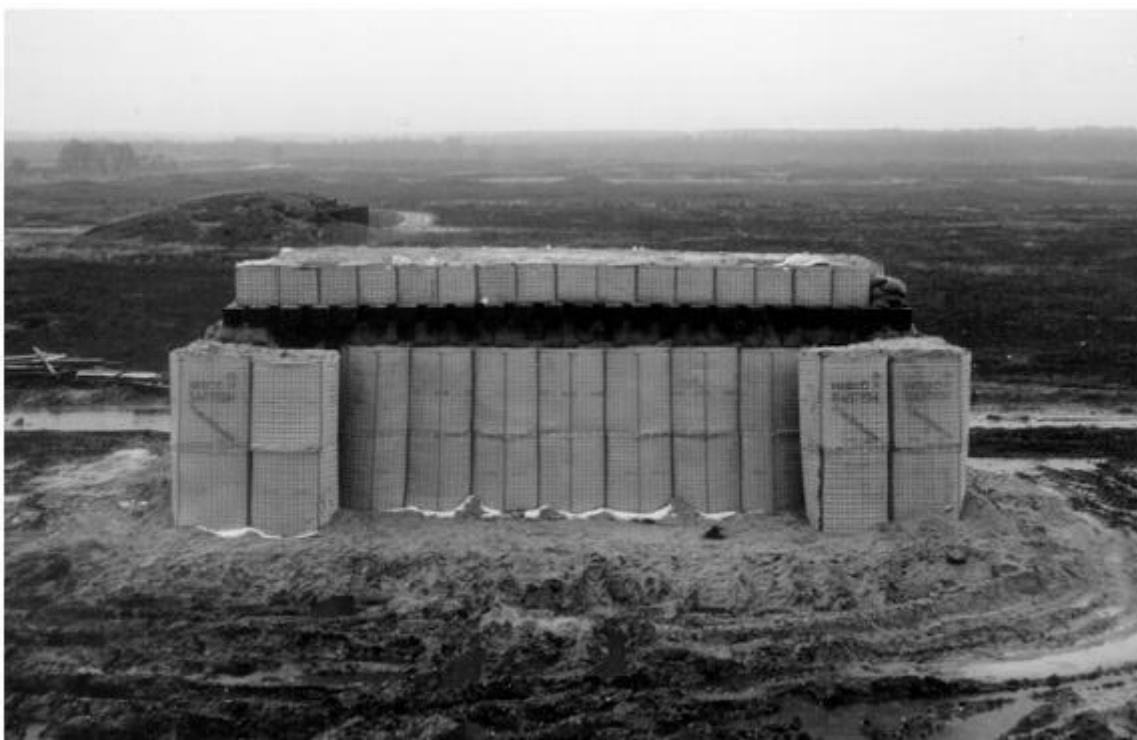
Figure 4H-2: Example of Protective Shelter
