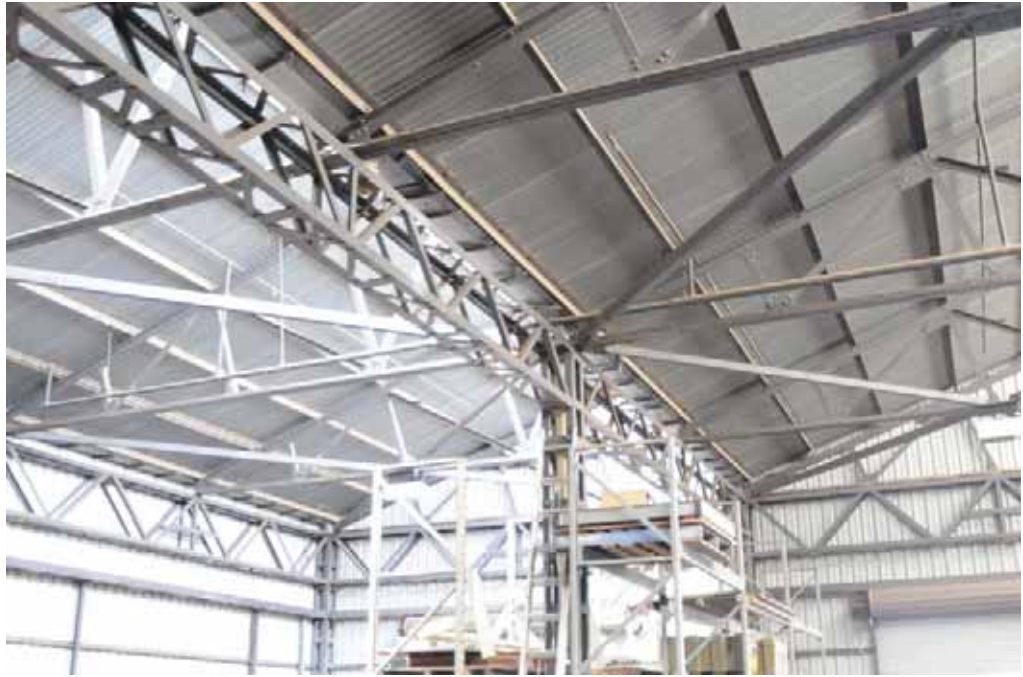
Figure 3.3 Interior steel frame detailing 26
