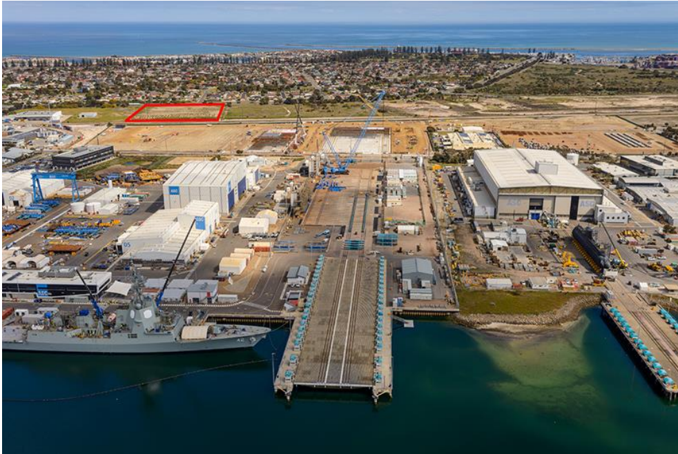
Figure 1: Osborne South Shipyard - aerial view
