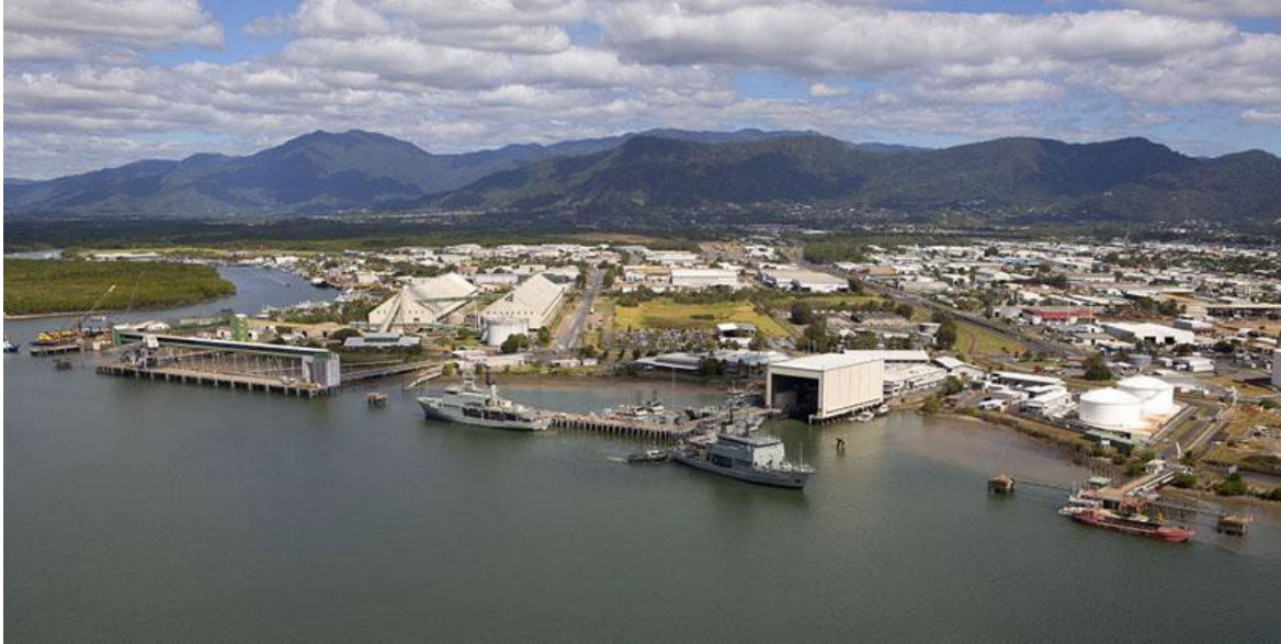
Figure 1: HMAS Cairns - aerial view
