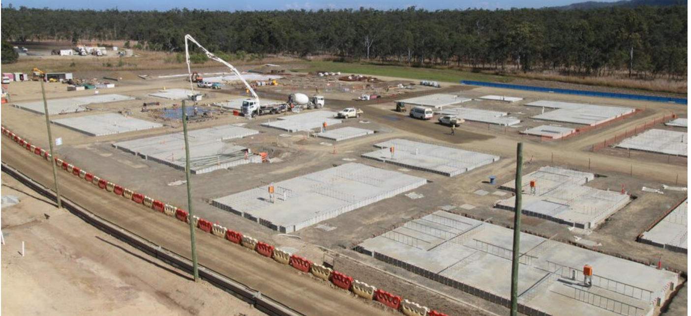
UOLF facility construction, SWBTA
