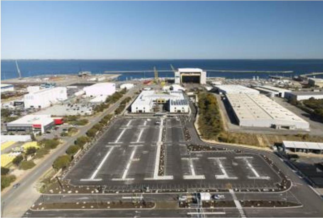
Figure 2: Henderson office accommodation
