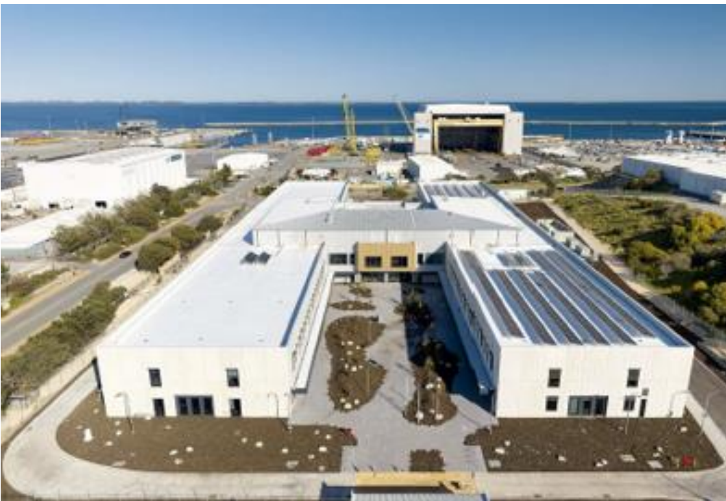
Figure 3: Henderson office accommodation
