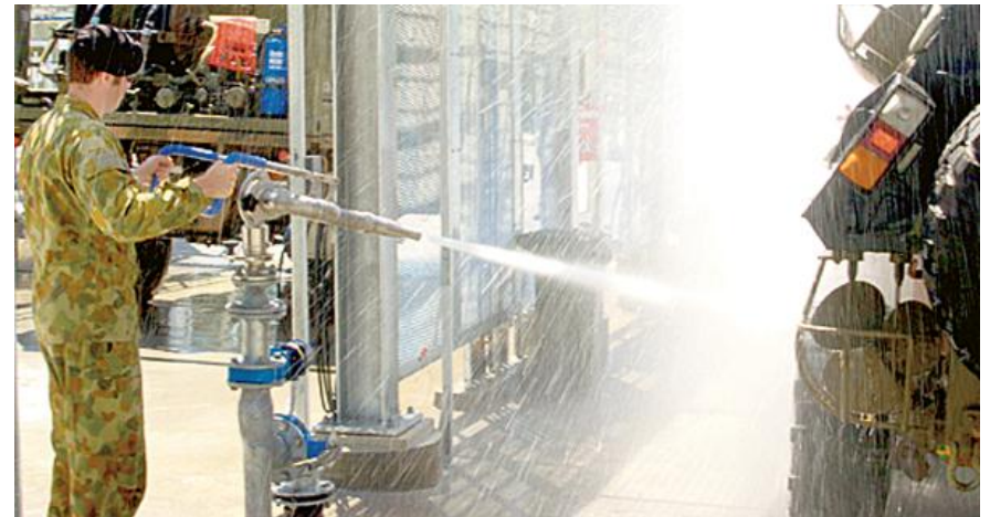
16-vehicle wash point, Enogerra, Gallipoli Barracks, Queensland
