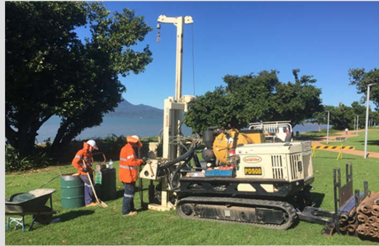
Small rig used to drill boreholes
