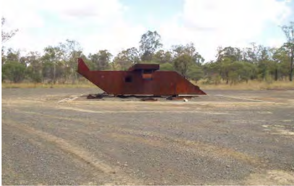
Figure 4.9. An example of a fire training facility at RAAF Amberley. The mock aircraft is on a porous fire tray (approximately 10m by 10m) that allows the collected foam water to drain into an underground pit. Any foam spray outside the fire tray remains in the environment.
