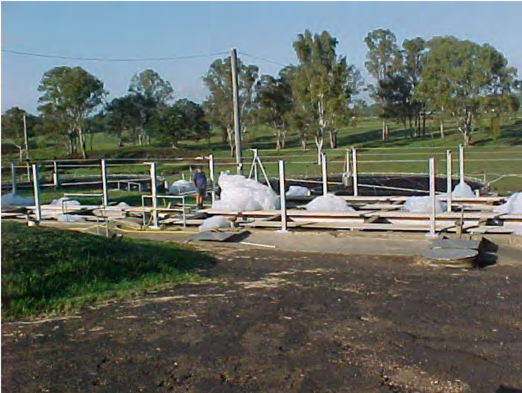
Figure 3.2. Excess foaming caused by AFFF waste at RAAF Amberley water treatment facility. (The excess foaming is not due to any fault of the sewage treatment plant operator.)
