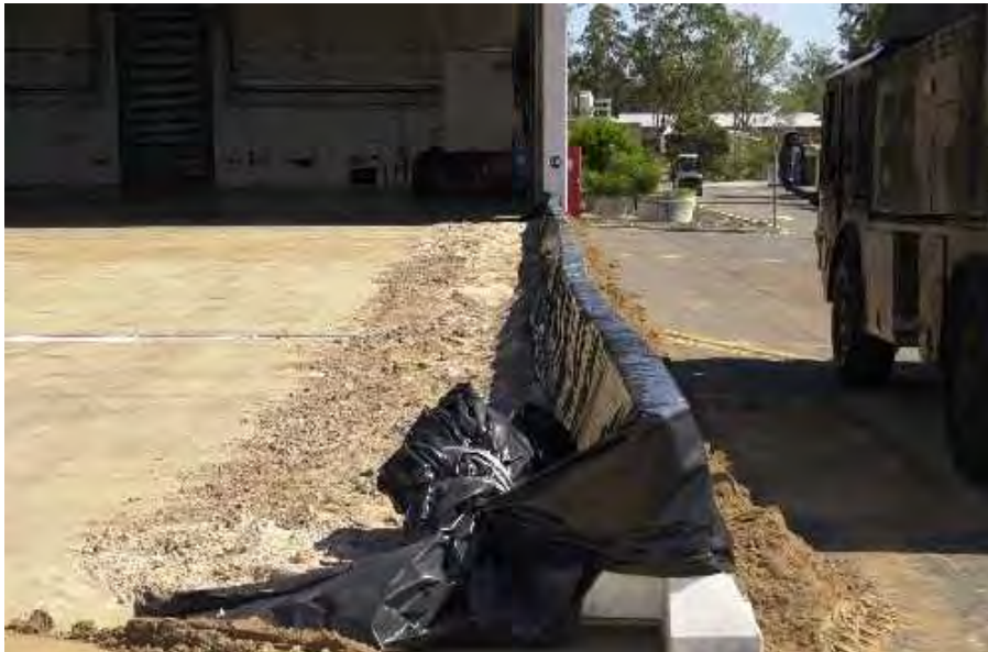
Figure 4.4. Temporary bunding outside a RAAF Amberley hanger in preparation of foam discharge during the testing of a hangars AFFF system.
