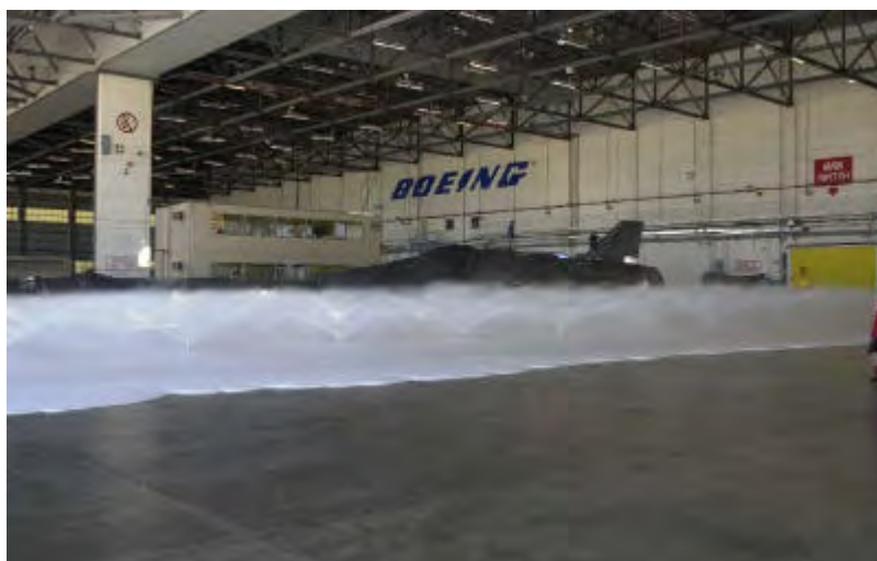
Figure 2.2. Activated AFFF foam sprinkler system test forming a foam blanket on the hangar floor.
