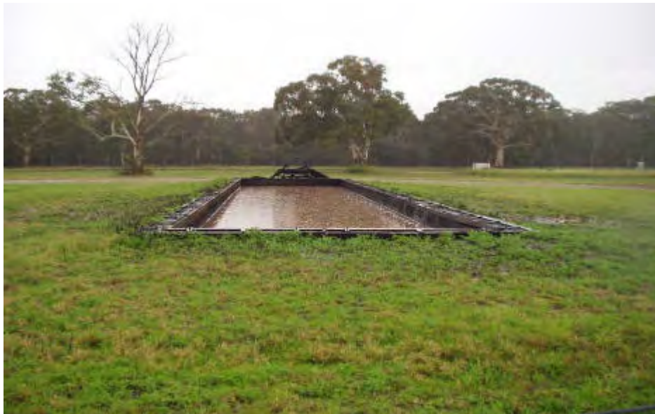
Figure 4.8. An example of a hot fire training pit at RAAF Williamstown. This pit does not have any controls to prevent spillage of fuel or AFFF flowing onto surrounding soil/grass areas.
