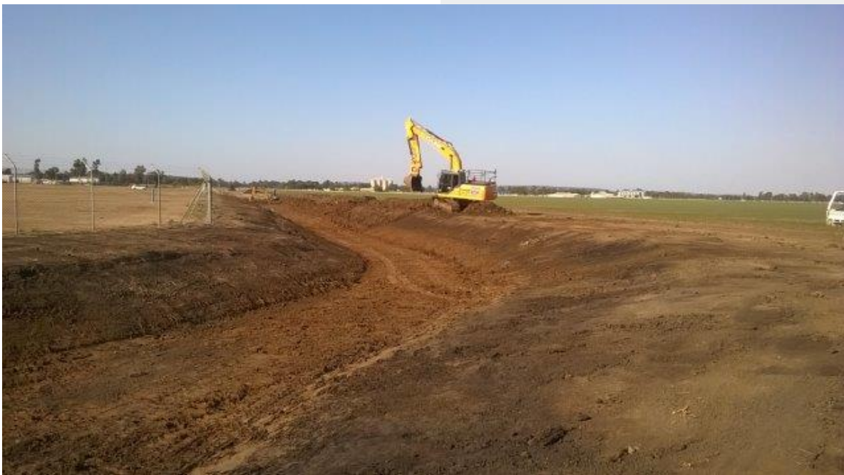
Below: Drain Maintenance Works
